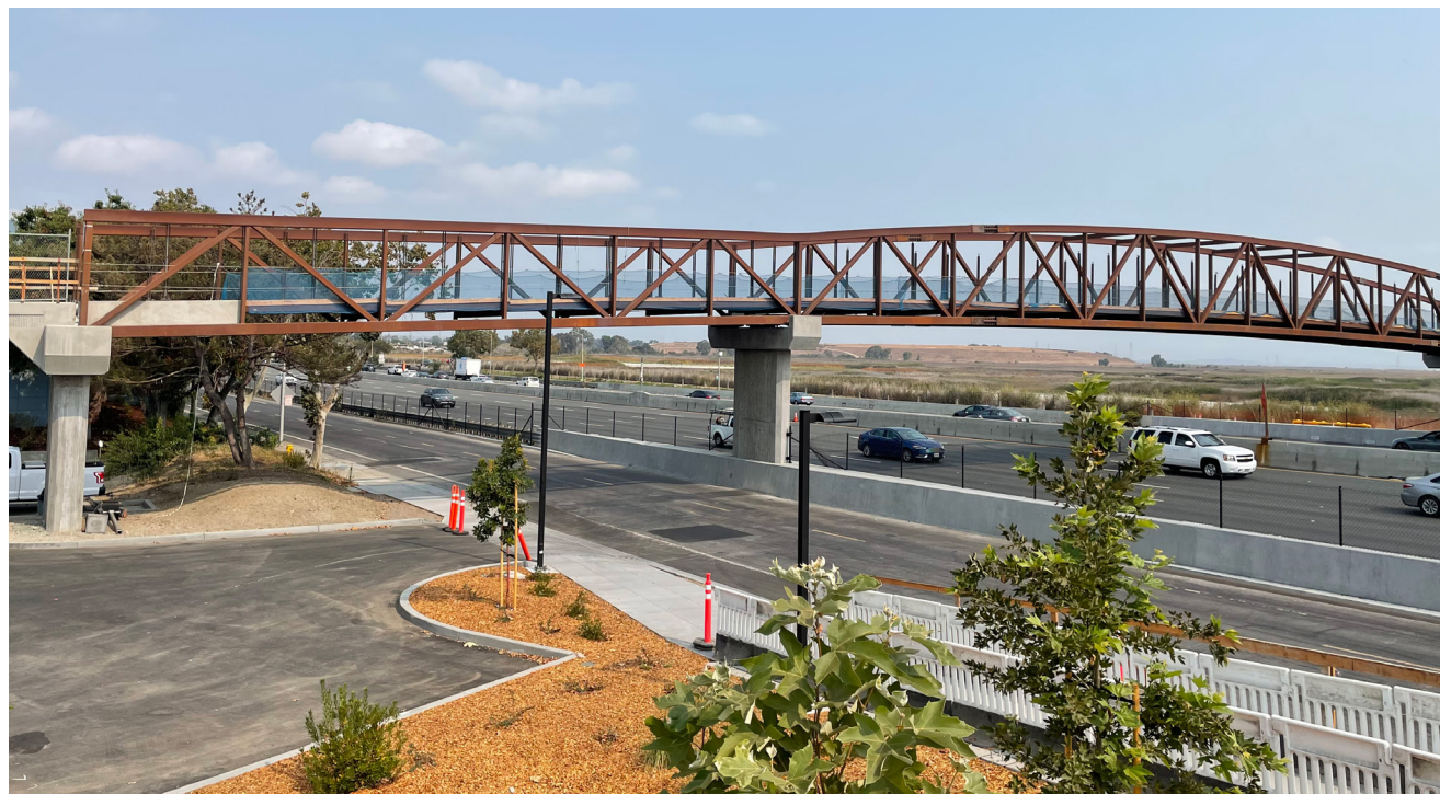
Adobe Creek Bike Bridge.
